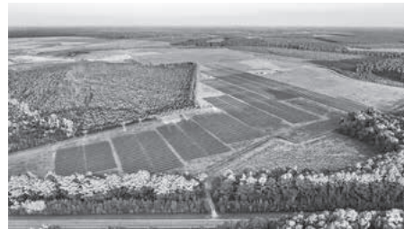
Solarpark „Aulander“ in North Carolina (7 MWp) – Renew Petra
